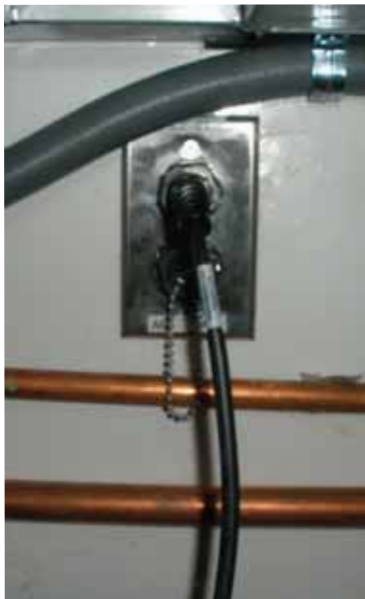
Siemon Ruggedized Z-MAX Category 6A shielded IP66/IP67-rated outlets and cords were deployed at Dodger Stadium's outdoor concession stands and kiosks
